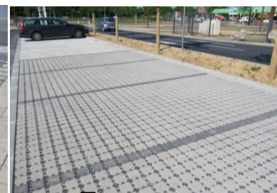
Pavés non jointifs joints
